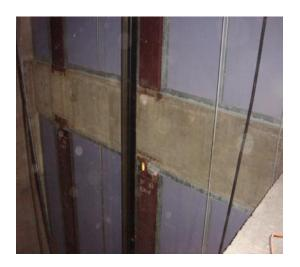
**Lesson Learned Statement:** Elevators ride up and down on guiderails that are located inside the elevator shaft enclosure. The National Fire Protection Association Life Safety Code, Section 8.6.5 requires shaft enclosure walls be constructed of a specific fire resistance rating to limit the travel of fire in a building.
